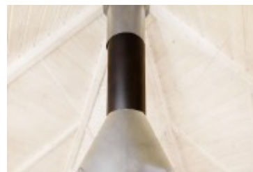
Grill Chimney Extension
