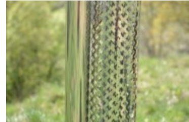
Metal safety fence for heater chimney
