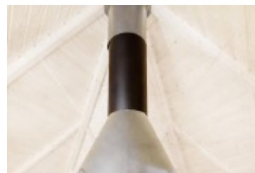
Grill Chimney Extension
