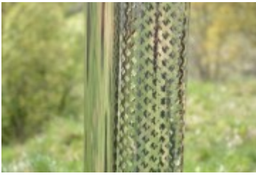
Metal safety fence for heater chimney
