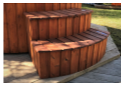
Stairs with niche for sand filter
