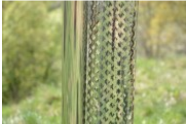
Metal safety fence for heater chimney
