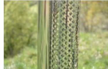
Metal safety fence for heater chimney
