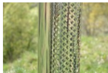
Metal safety fence for heater chimney
