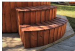
Stairs with niche for sand filter
