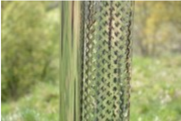
Metal safety fence for heater chimney
