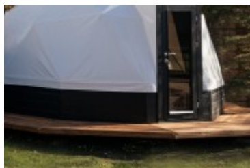
Terrace floor segments
